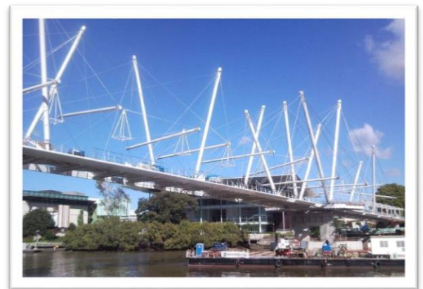
Photo : pont Kurlipa (Cox Rayner, 2009)
